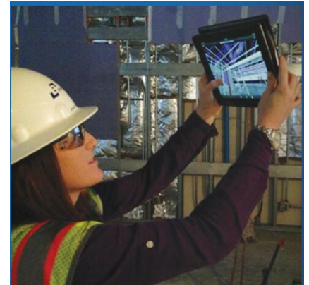
Figure 16 BIM 360 Field sur le chantier (Source : https://www.qualityinconstruction.com )
